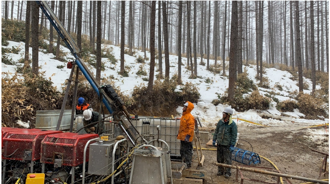
Figure 10-3: Ranger Series 4 Drill Rig, Drilling KT19-02A
