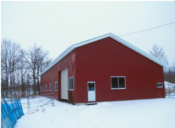
Figure 12-2: Core Storage Facility, Kato Property
