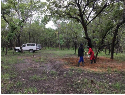
Plate 2.6.1: Overview on CT1 position post rehab.
